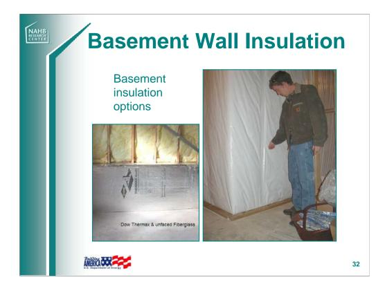
Continuous insulation is an important detail when insulating foundation walls.
