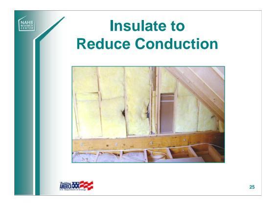
Insulation helps slow the flow of heat into and out of a home.
