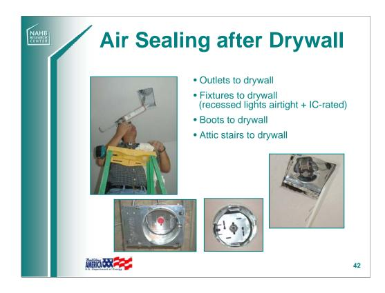
Air sealing from the interior, or finished side, of the living space can help to reduce air leakage into or out of the home.
