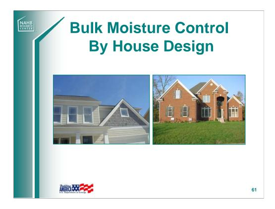
When roofs direct water toward sidewalls or adjacent roof areas the potential for water intrusion grows.
