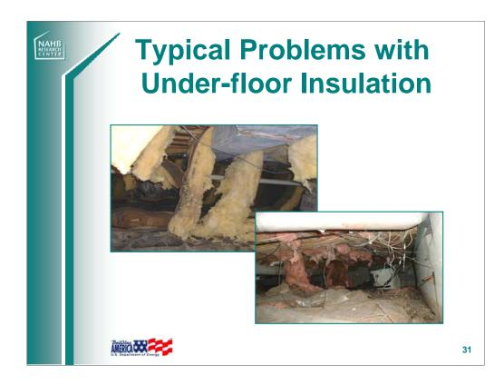
Floor cavity insulation has to fight gravity to stay in place, and be tight against the subfloor, in order to be effective.
