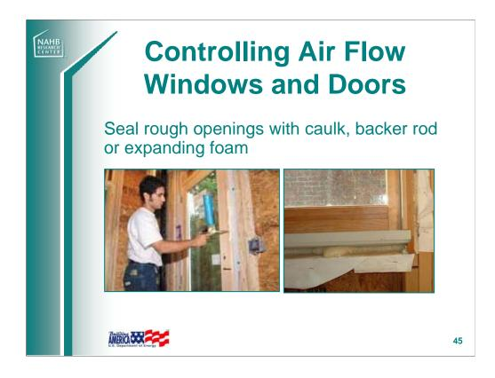
The joint between window and door frames and the rough opening can be a major source of air leakage.
