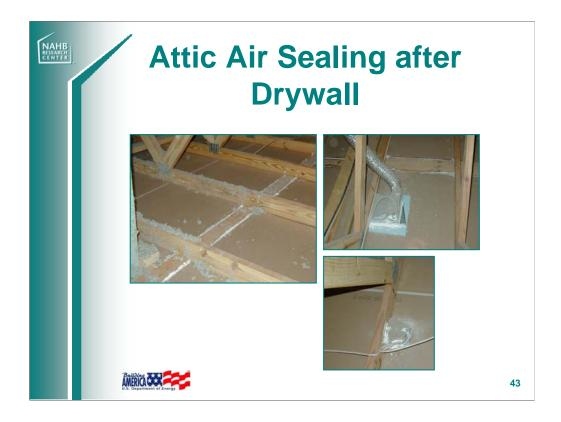
Air sealing from the attic, prior to insulation installation, can be easier than from interior.
